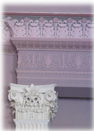
No. 13 First floor cornice
