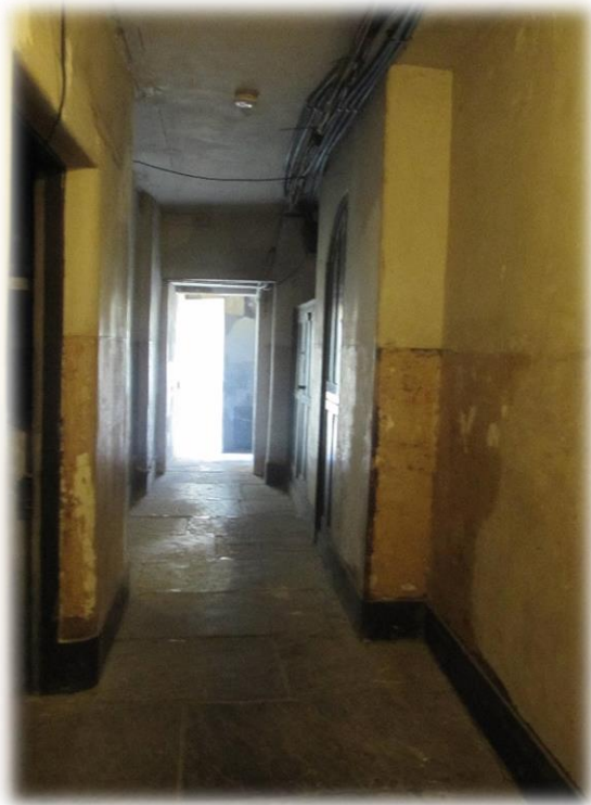
Hallway of No. 10
